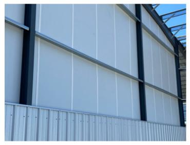
Steel Stud Wall Construction TSX-8510 // Exposed Interior Use & Quick Clip // Insulation Attachment System
