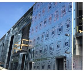
Steel stud framing with 2" ECOMAXci® FR Air Barrier attached directly to the studs. R-SEAL 3000-4 tape and R-SEAL 6000-9 flashing. The facade was a combination of stucco, brick veneer and ACM metal panels.
