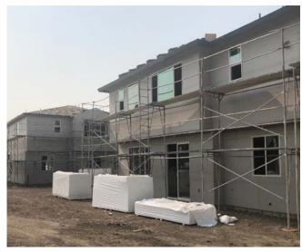
Open stud wood framing (except at structural/ shear conditions) 2-ply 60 minute asphalt saturated paper, 1" Rmax polyiso insulation with drainage mesh facers, lath, 1-coat stucco
