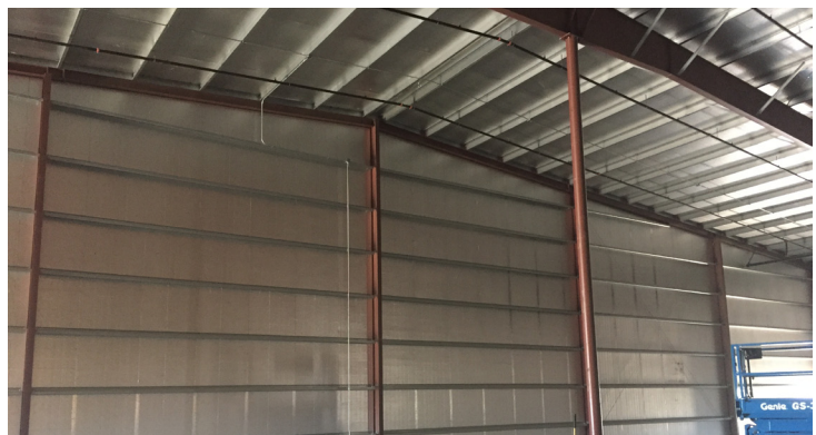
Metal building construction with Rmax ECOMAXci® FR exposed insulation.
