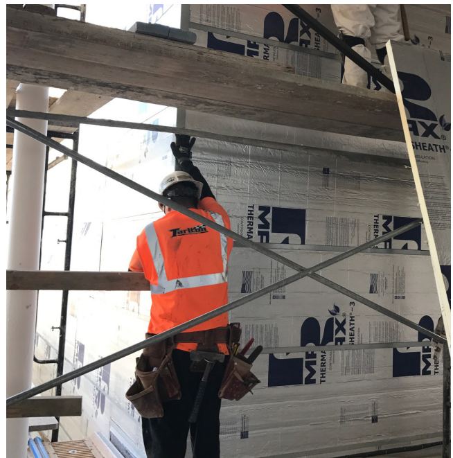
Thermasheath® over exterior gypsum installed between Z girts.
