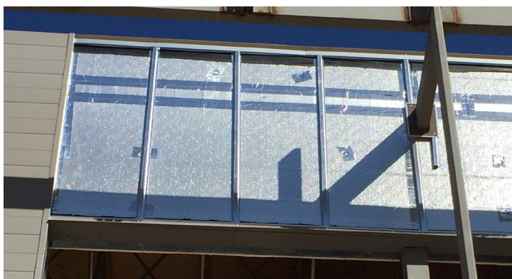
Steel stud construction with Rmax TSX-8500 and a metal panel facade
