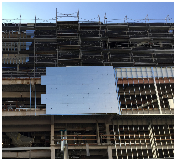
Steel stud construction with Rmax ECOMAXci® FR
