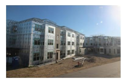
Rmax ECOMAXci® Wall Solution includes a thermally efficient continuous insulation board and Rmax branded tape and flashing. This solution has been tested in multiple NFPA 285 assemblies and is approved for use in exterior walls of buildings of any height.
