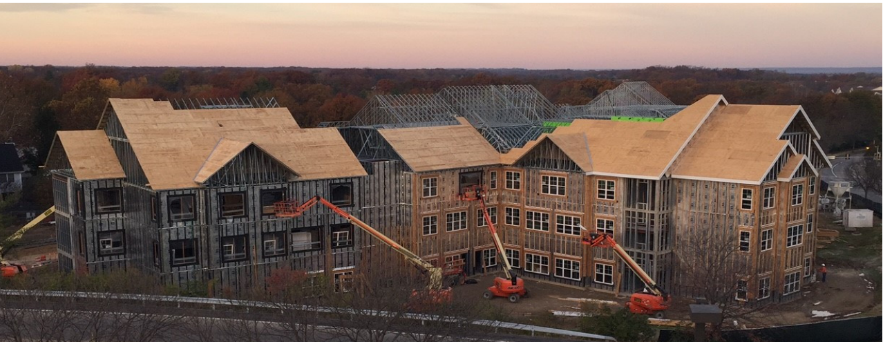
Assembly: Steel stud
