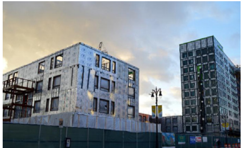
Assembly: ECOMAXci® Wall Solution attached to steel studs. Masonry façade. ACM/MCM façade.
